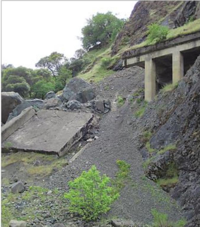
The tunnel immediately south of the Woodman Creek crossing has collapsed and been partially filled by one of many landslides exacerbated by the defunct rail line in the Eel River canyon. Photo: Scott Greacen.
