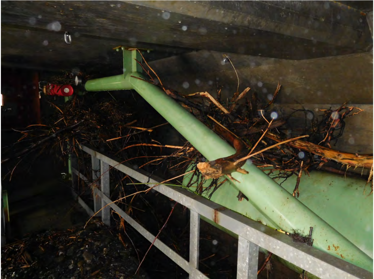
Woody debris in the upper portion of the fish hotel structure.
