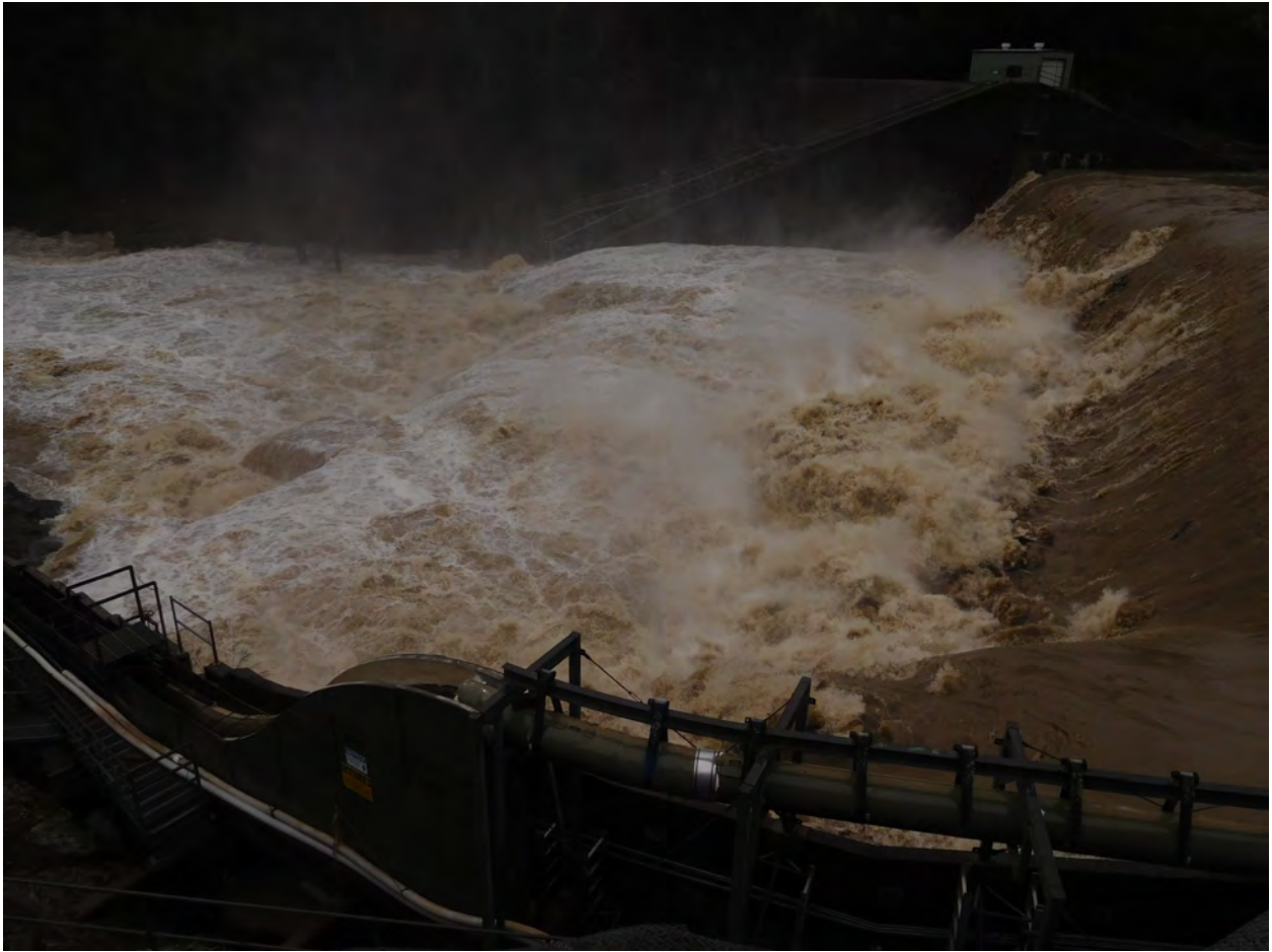
Cape Horn Dam with the Eel River flowing at approximately 16,400 cfs.
