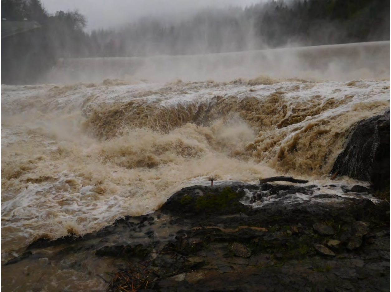
Cape Horn Dam with the Eel River flowing at approximately 16,400 cfs. The 'fish hotel' structure is entirely underwater in the center-left portion of the photo.
