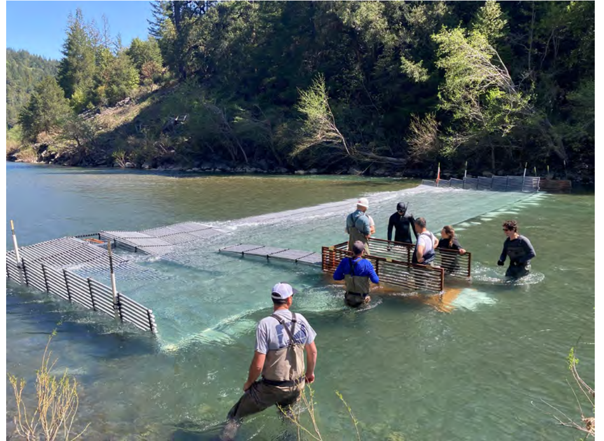
South Fork Eel River Weir for Pikeminnow Suppression, April 25, 2023
