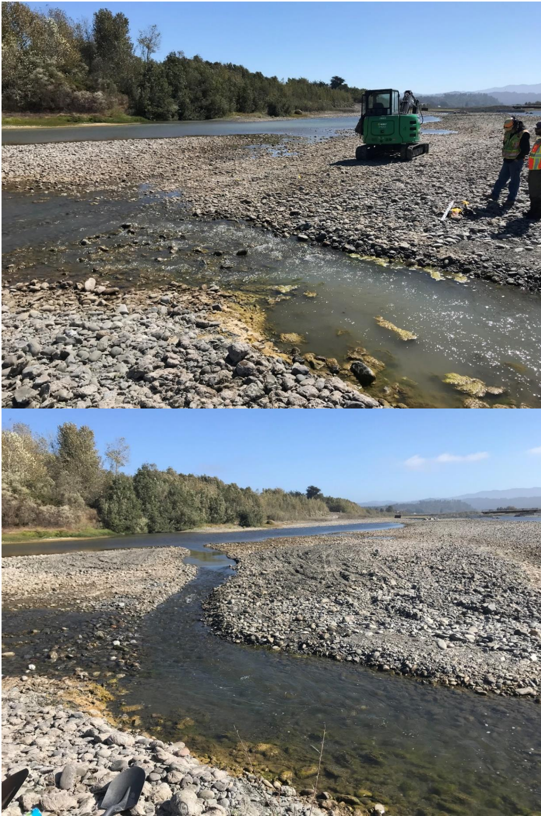
Figure 2. The constructed riffle prior to alteration on September 15, 2021 (top) and after alteration on September 16, 2021 (bottom). This constructed riffle provides a strong downstream flow-signal, a riffle depth ranging from 10 – 15 cm, a recovery basin with a max depth of 44 cm, and a riffle crest depth of 15 cm. Initial measurements indicate upstream pool depth was successfully maintained.
