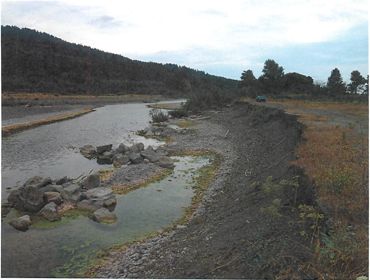
Figure 2: Unauthorized revetment structures along the bank of the Van Duzen River at the Project site, now in the active channel of the Van Duzen River, July 2015.
