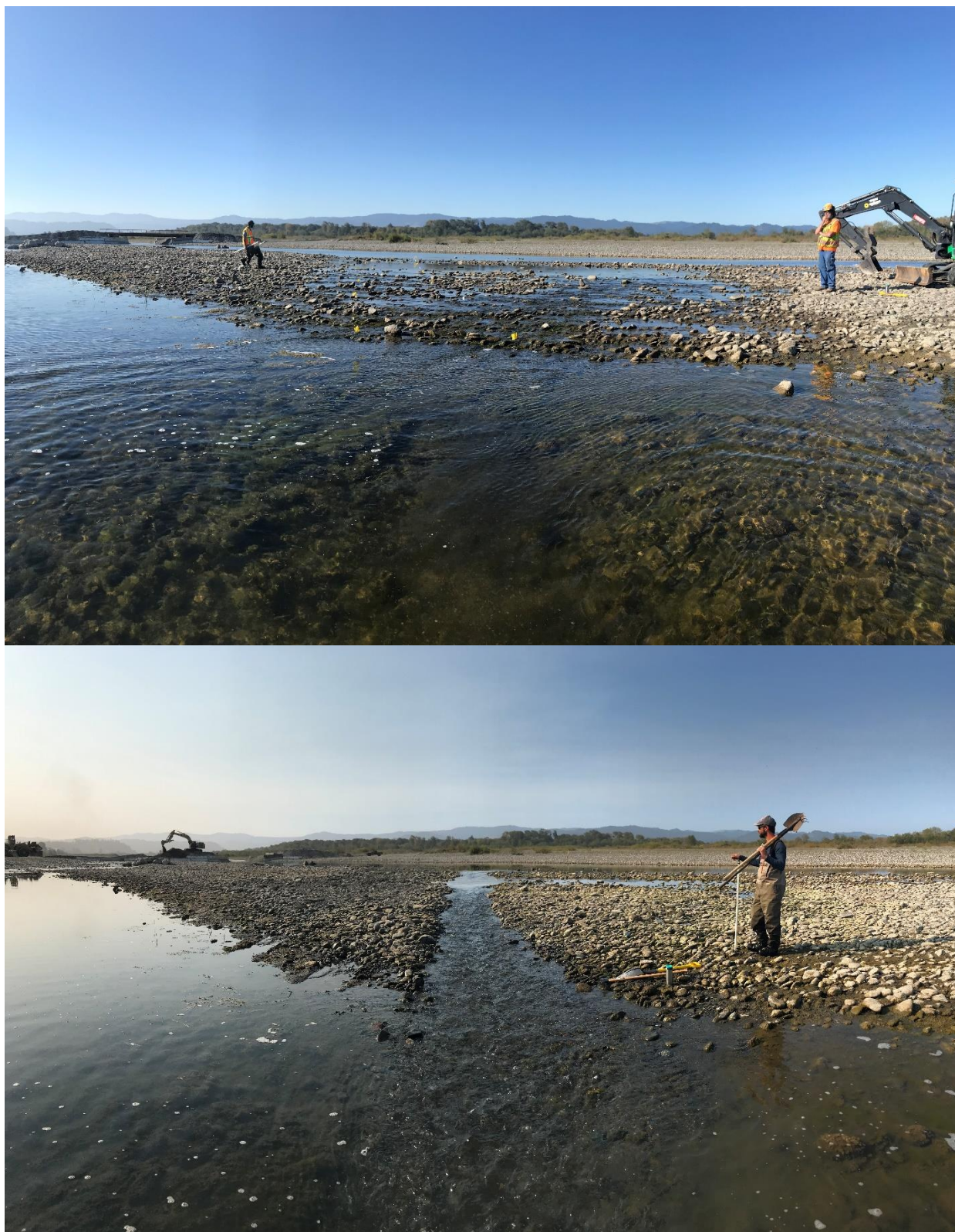
Figure 1. Riffle D prior to alteration on September 15, 2021 (top) and after alteration on September 16, 2021 (bottom). The altered riffle provides a strong downstream flow-signal, a riffle depth ranging from 10 – 15 cm, a recovery basin with a max depth of 56 cm, and a riffle crest depth of 11 cm. Initial measurements indicate upstream pool depth was successfully maintained.
